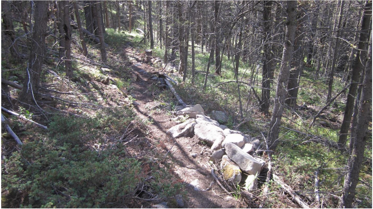
Figure E17. Trail cut into the ground and cleared of trees and rocks.
