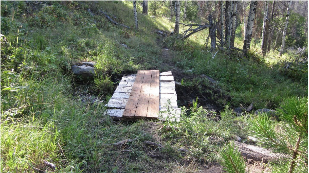
Figure E24. Shorter bridge than Figure E23.
