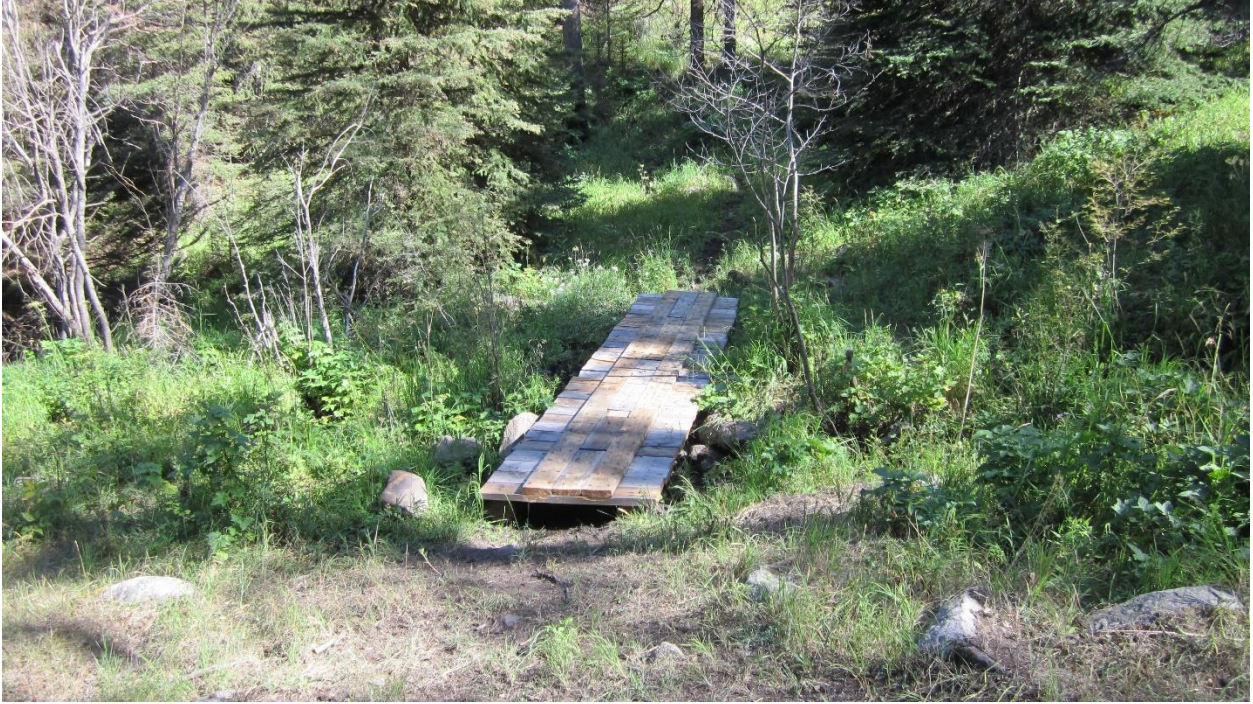
Figure E23. Long wooden expanse placed along illegal trail crosses stream riparian area.
