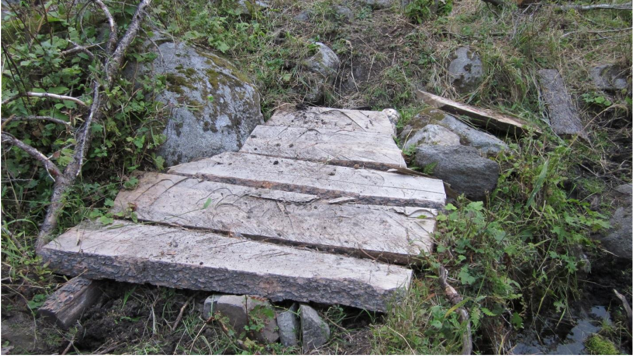
Figure E25. Wooden planks put into a boggy area.
