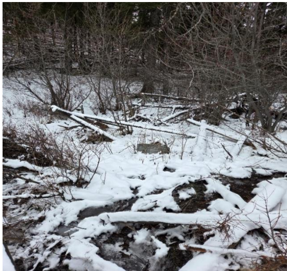
Figure E10 . Existing tanks are in good condition. 46.53340 -112.20352
