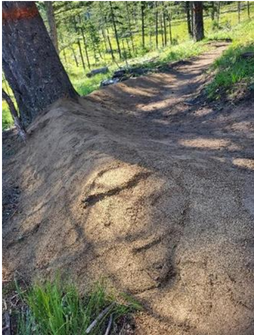
Figure 24. Banked trail recently constructed in Travis Creek
