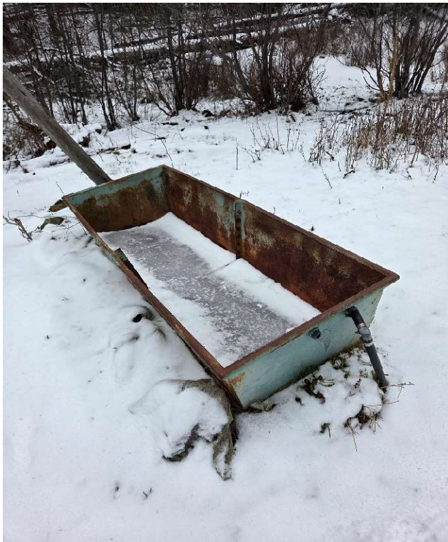
Existing Tanks are in Good Condition. 46.53340 -112.20352
