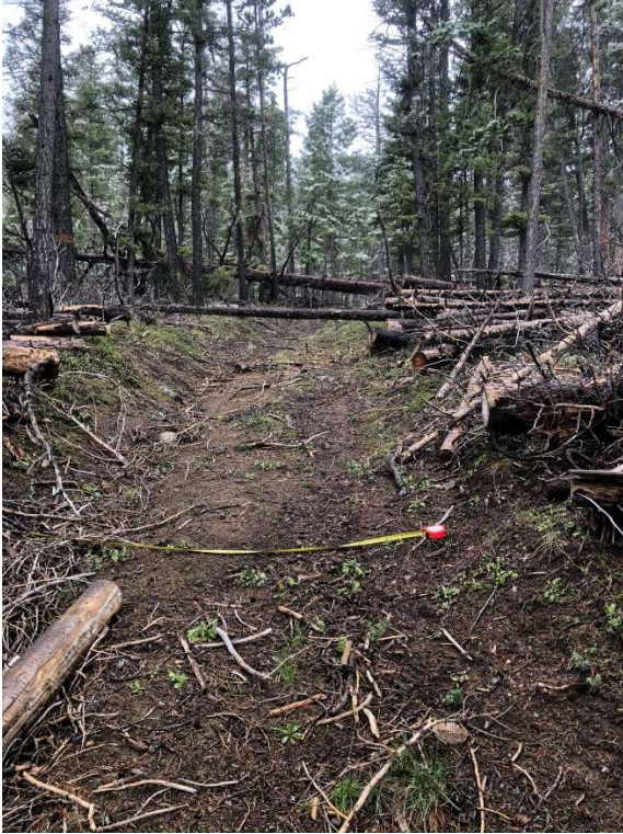
647-NS15-7 Looking south. The road on the transportation map is only a trail. This is the actual road. 6-8' wide. 5-10% slope.
