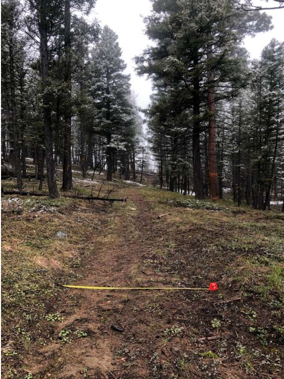
647-NS15-9 Looking south. Trail cleared of blowdown. 8' wide 10% slope.
