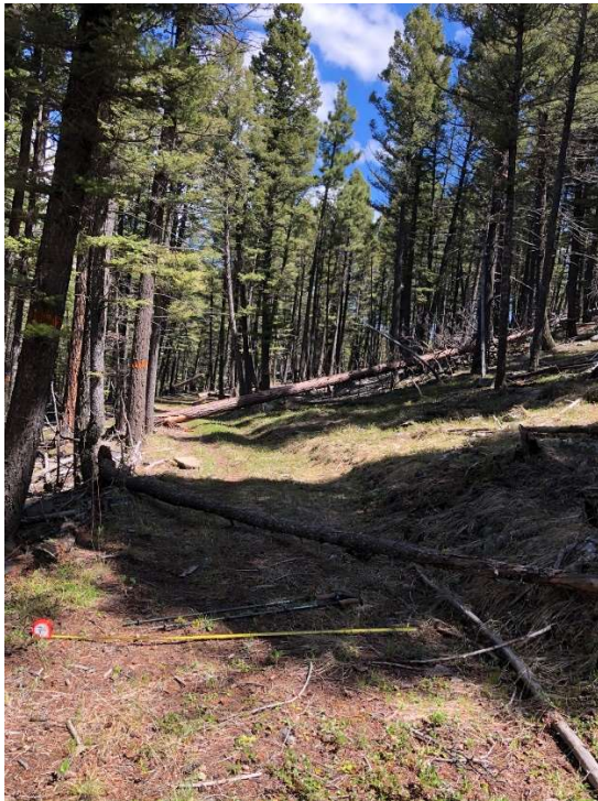
647-NS09-4 Looking back. 7' road bed. Some blowdown. Map road does not align well with actual road. Larger firs – some painted orange. This is proposed regeneration harvest unit 102.
