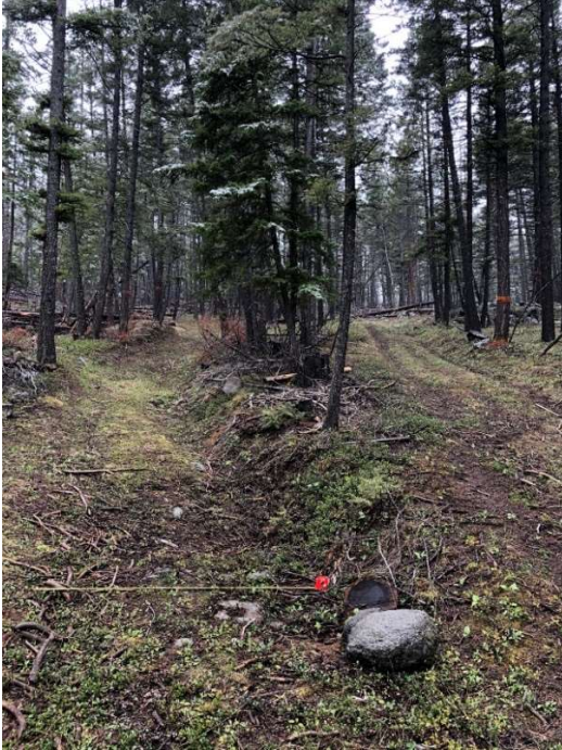
647-NS15-1 Start of NS15 spur road, starting from north end. 6-7" wide. 10-15% slope.
