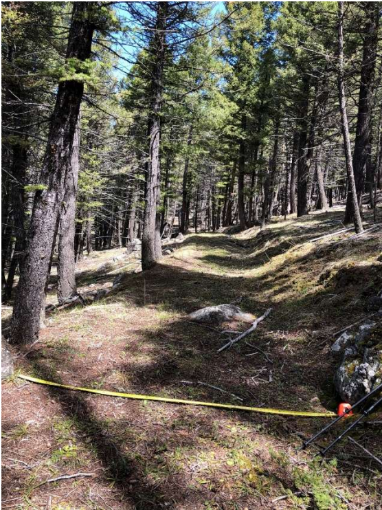
647-NS09-14 Coming back down. Showing roadbed width 7'. Flagging of trees ends about 100 yards before the road turns to a trail.
