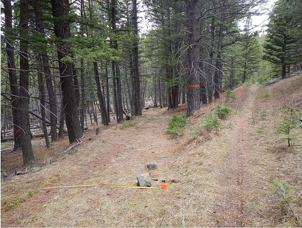
Waypoint 27.1 #4000.NS01 goes right and #4000-NS04 goes left. Looking southwest. Tape = 6'. 25% slope. Seedlings growing in old roadbeds.
