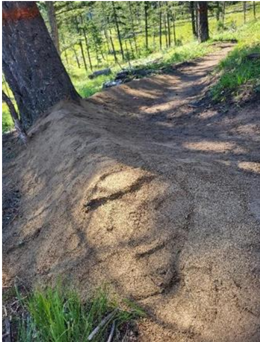
Figure 24. Banked trail recently constructed in Travis Creek
