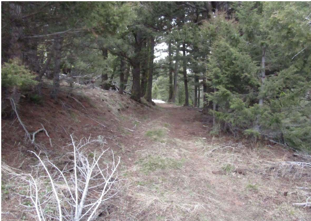
WAYPOINT 007 - Road bed encroachment by lodgepole pine, Douglas fir, and ponderosa pine regeneration, mature Douglas fir on sides of road bed, north photo direction, 12-15 foot road width.
