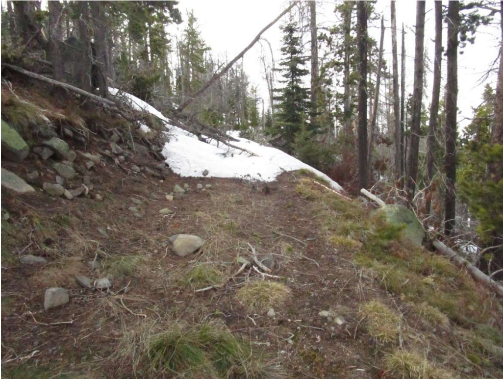
WAYPOINT 010 - Old road bed, some large rocks, wind blown dead fall and snow, NW photo direction, 8 foot road width.
