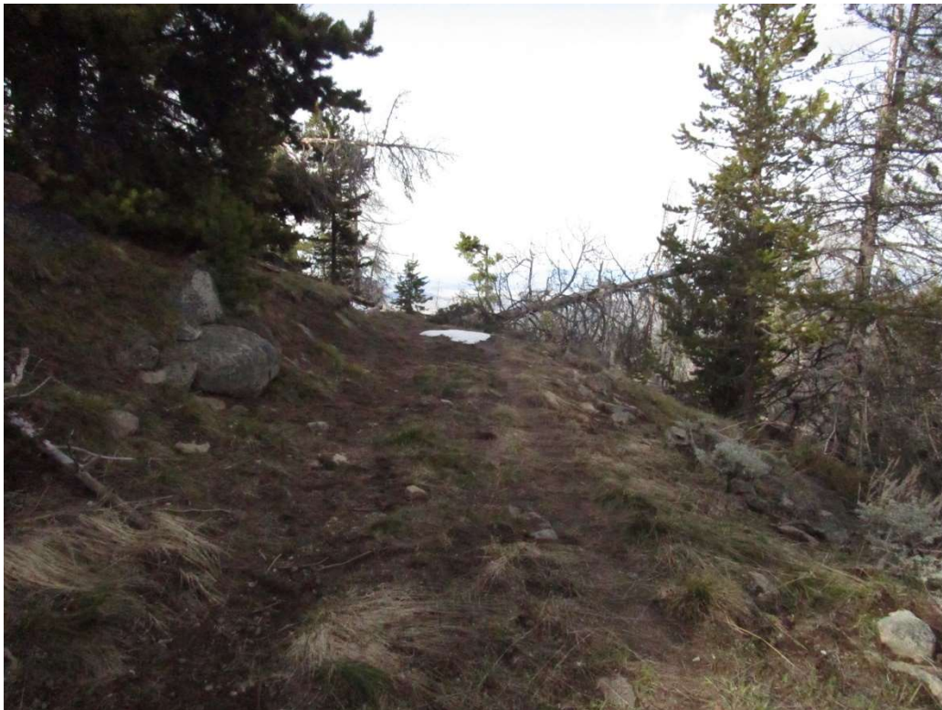
WAYPOINT 009 - Old road bed with lodgepole and Douglas fir saplings, some large rocks on west side of road, NE photo direction, 8-10 foot road width.
