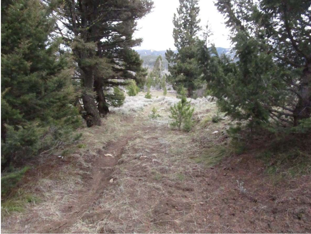
WAYPOINT 007 – Road bed encroachment by sagebrush and lodgepole pine, Douglas fir, and ponderosa pine regeneration, south photo direction, 12-15 foot road width.
