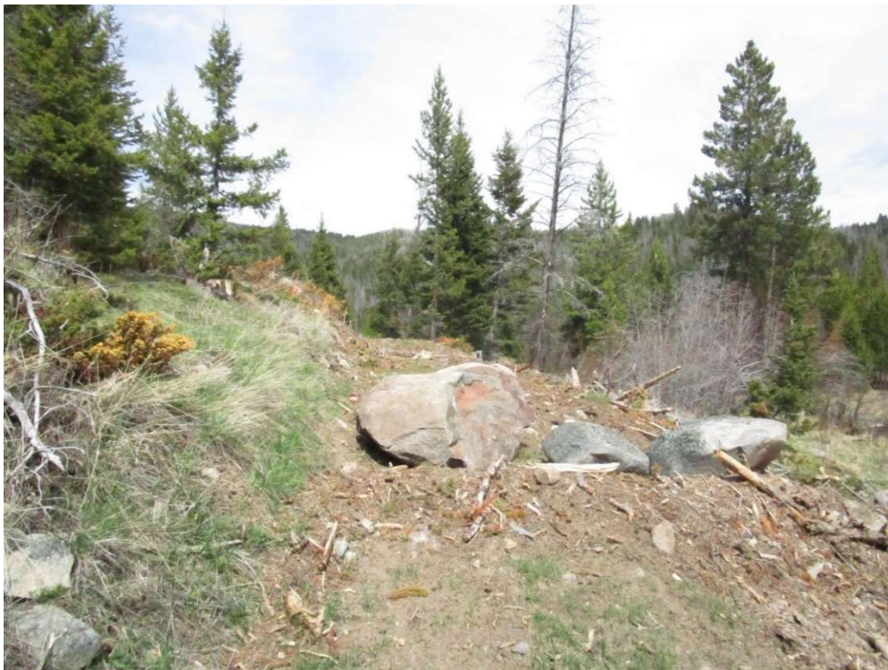
WAYPOINT 012 – Start of 299-NS05. Large rock road blocks used. Road development with woody debris due to recent timber harvest, NE photo direction.
