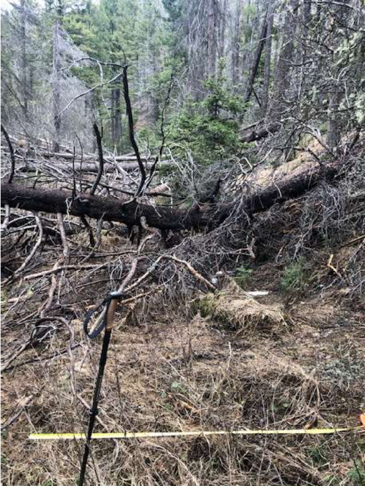
PHOTO NS03-3. Approximately 300 feet further down the road showing extensive blowdown on the roadbed. Tributary creek is on the left side.
