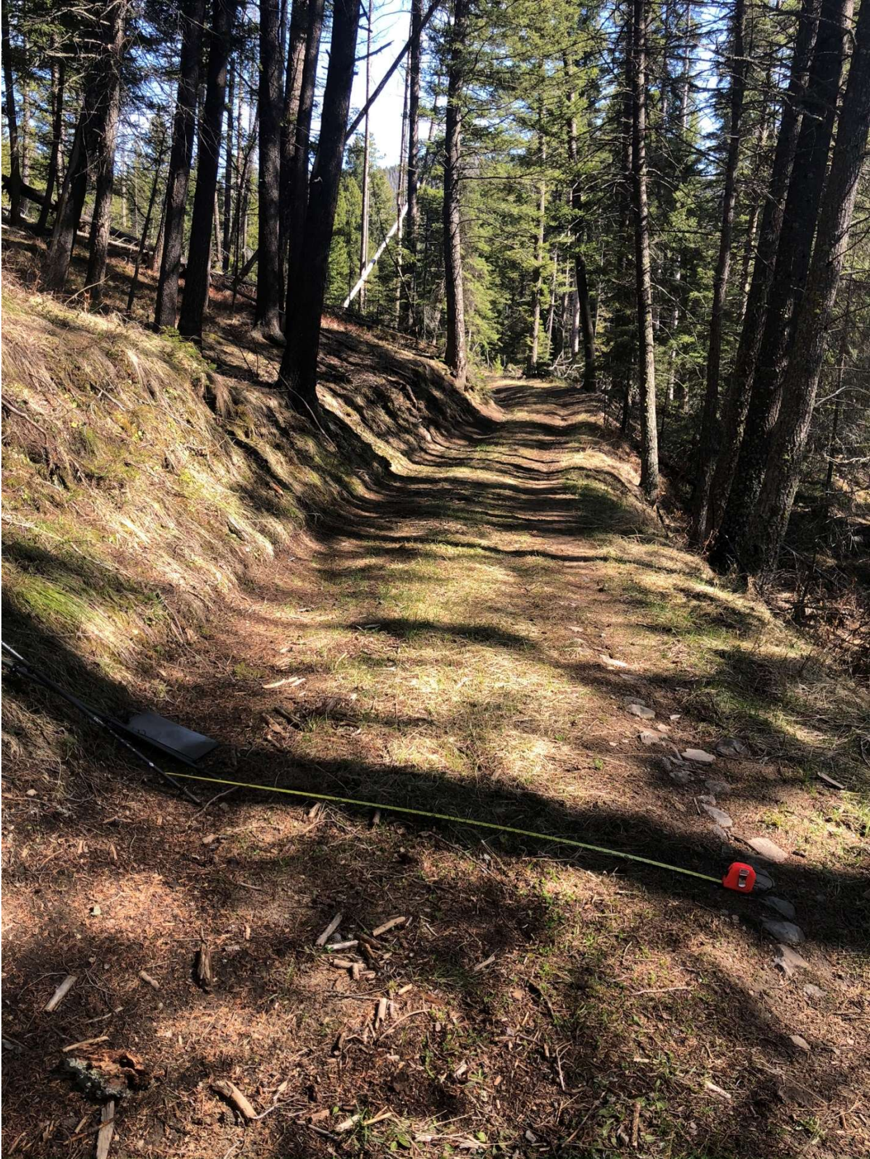
PHOTO NS01-3. 300 feet further up the road in the direction of travel. 7-8 foot roadbed.
